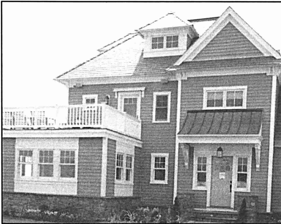
IDEA COTTAGE – The exterior of the cottage is finished with synthetic materials designed to look like a real Maine cottage without all the maintenance wood requires. At left, the living room on the first level of the cottage has furniture surrounding a gas fireplace. The French doors lead out onto a patio, where there is an outdoor fireplace. (Emma Bouthillette photos)
